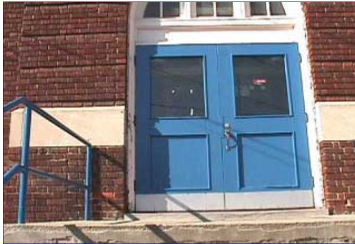
Concrete repairs required for the southeast stair
