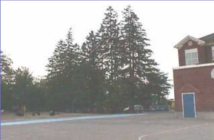
There is only some minor cracking on all paved areas
