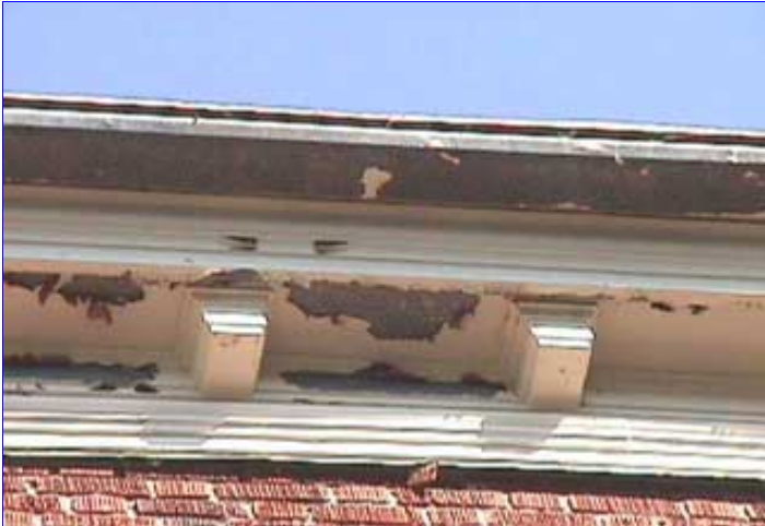
The main building gutters require repairs and new down spouts
