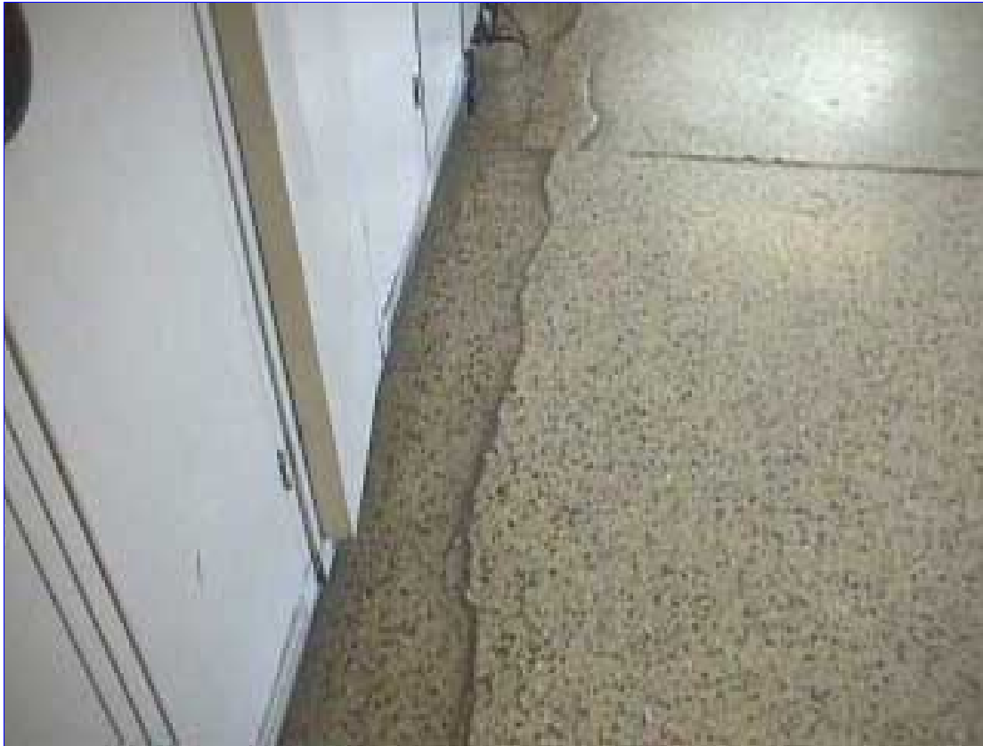
Settlement cracking in the terrazzo floor of the annex
