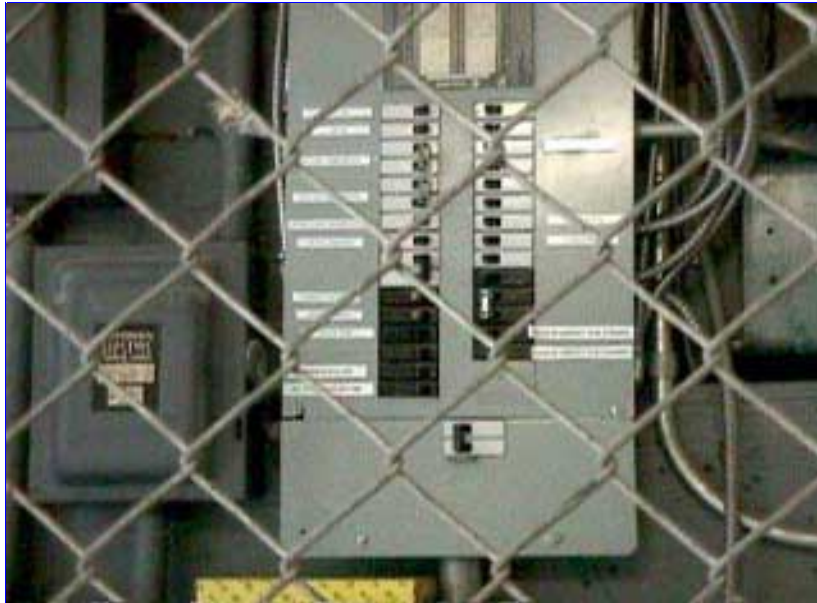
The panels and boxes have new breakers and fuses
