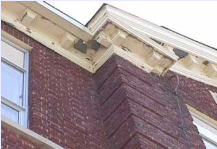
The painting of the main building soffit and fascia is in poor condition
