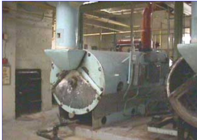
The existing boilers have just been re-cored
