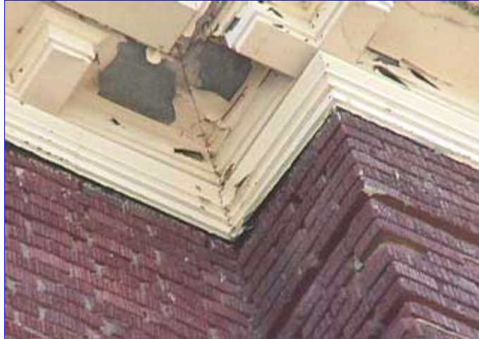
The exterior is in need of painting
