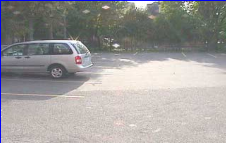
The parking area was repaired last year
