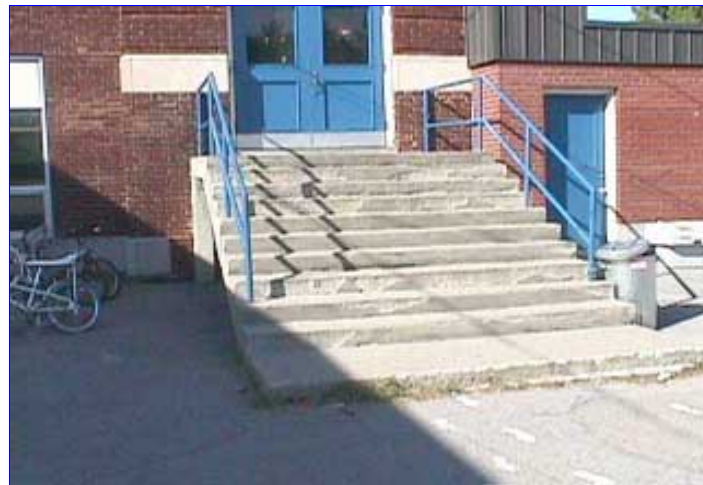
The spalled concrete is a safety hazard
