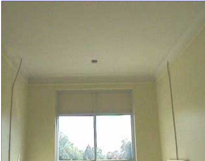
The plaster walls and ceilings are in remarkable condition
