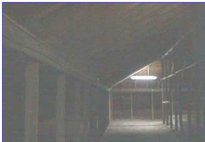
The wood frame structure of the existing building roof which is in excellent condition
