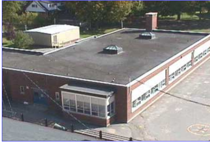
Roof of the annex
