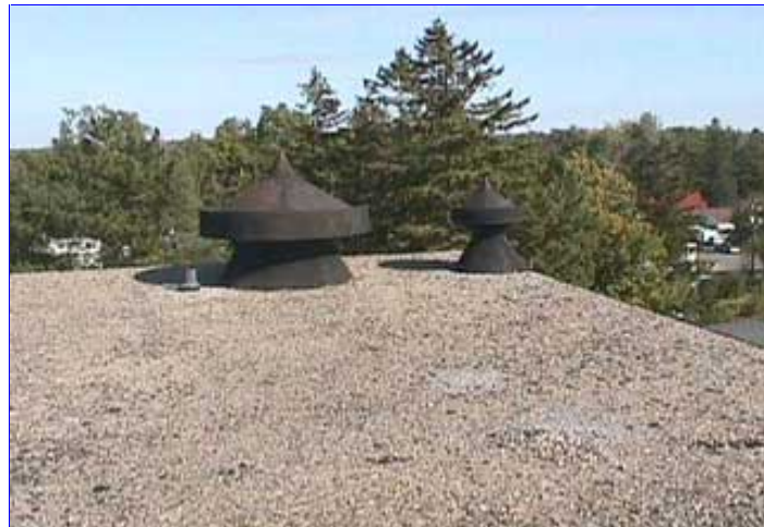
Flat roof area of the main building
