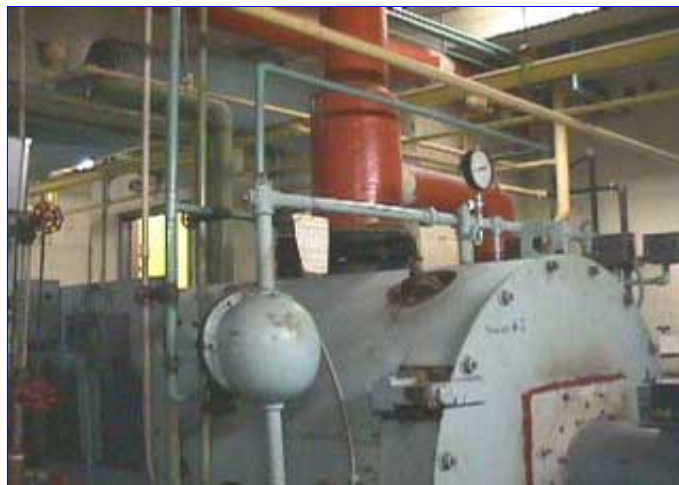
The piping and pipe insulation is in good condition
