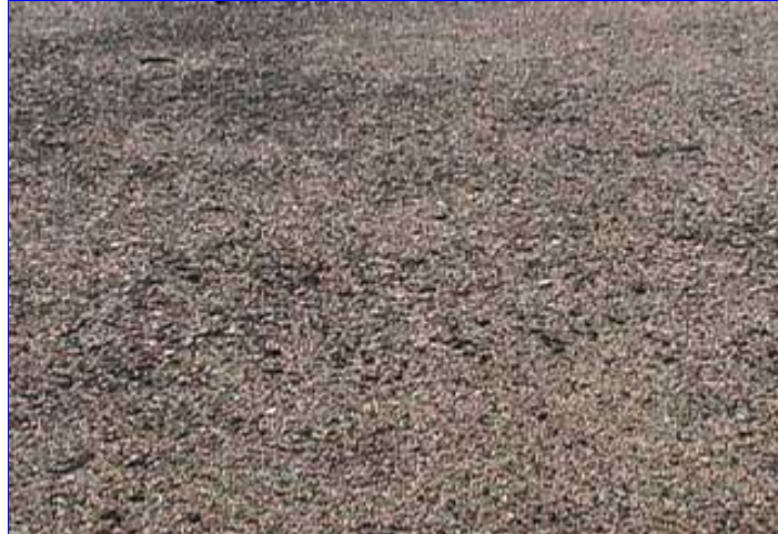
Built up roof has only minor blistering
