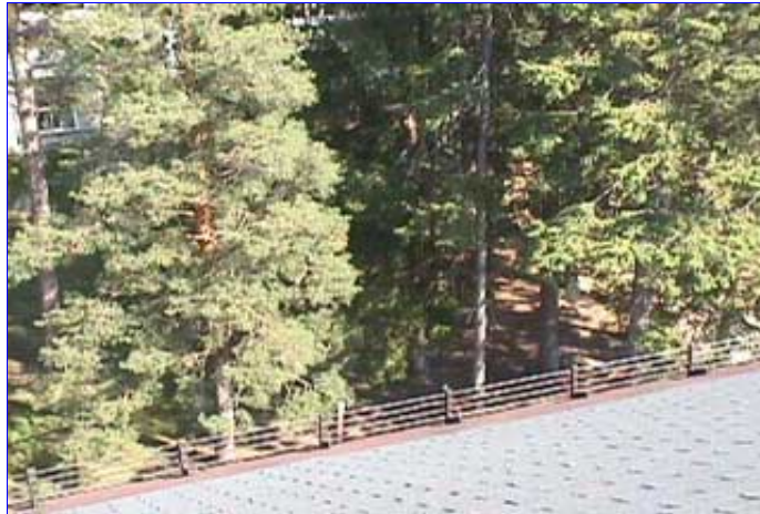
Main building – shingled roof with ice fence around the perimeter
